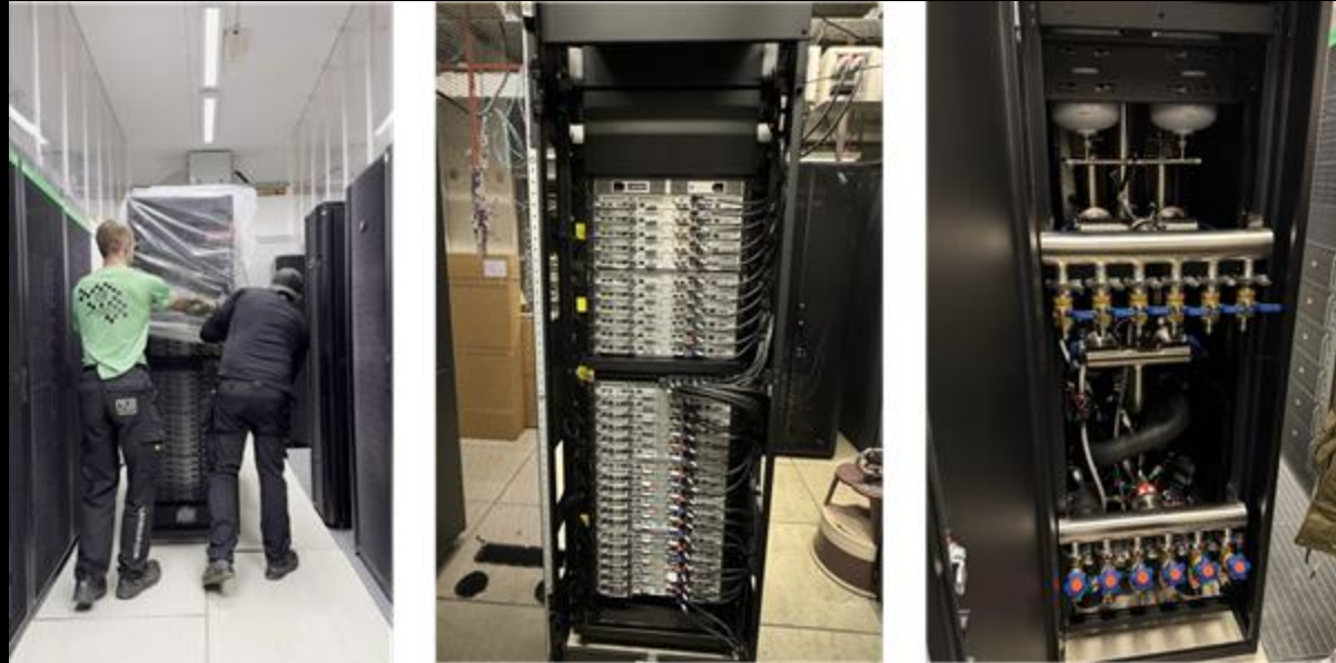
60 nodes (30 trays) of SD665 V3 with 2 x 9654 CPUs
